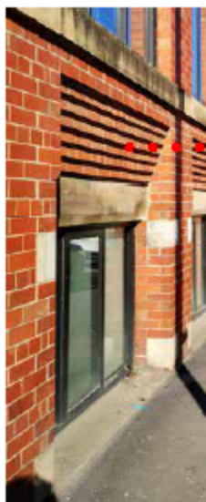
Brick detailing to openings - Britannia Mill
